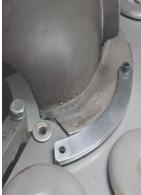
Use broken corners for shims or use washers lower than remaining plate height. Grind plate weld or strap for clearance before securing.
