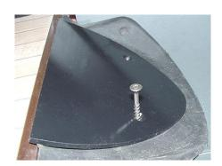
For best results, insert and seat screw vertically to apply downward force to starter block and SBR to keep reliable permanent positions. The hole countersink is merely to improve mounting results as compared to results of providing holes not countersunk.
