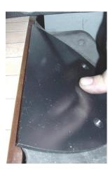
CAUTION; Avoid over tightening of fasteners to prevent hole stripping in plastic and wood gutters.
